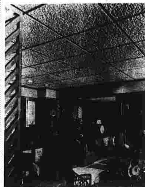
TRIED-AND-TRUE RECIPE for decoratively uniting the cooking and dining areas of an eat-in kitchen is the installation of a striking ceiling. The 2' x 2' panels of this Armstrong suspended ceiling descend slightly below the supporting grid for a bold-relief effect.
